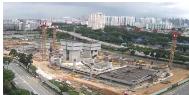
Super structure work in progress for Block 1 and Block 2. Completed piling works for Block 3
